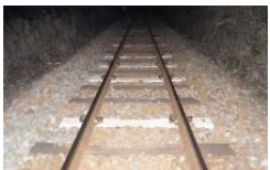
Transitioning to TPC railroad ties
