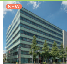
NEW Hakata Chikushi-Dori Center Building
